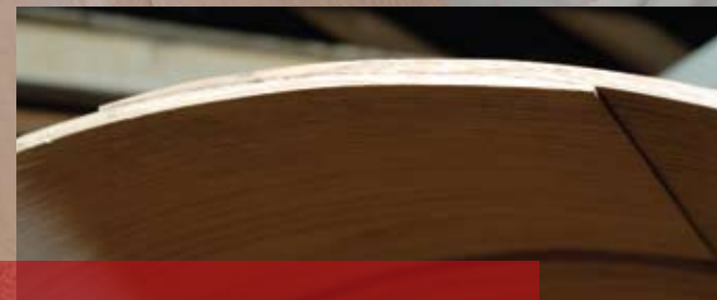
A close up view of the scarf joint of the shell.
